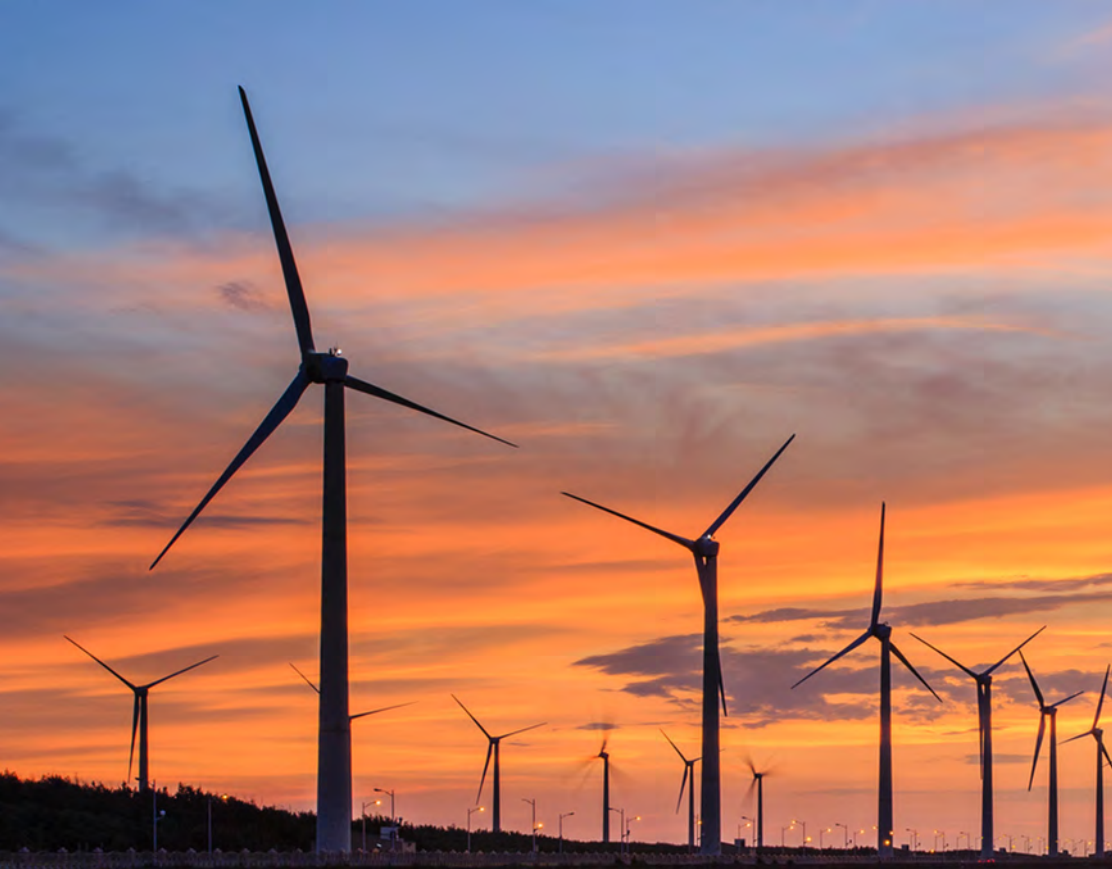
Autotex wind farm at Karnataka - India
