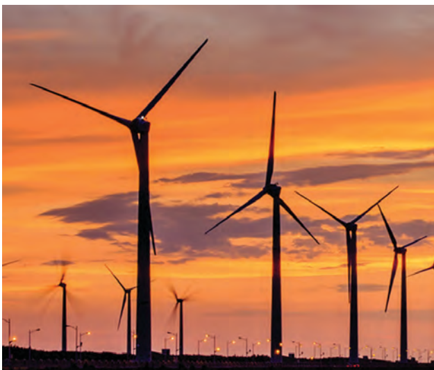
Autotex Believes Green Energy
