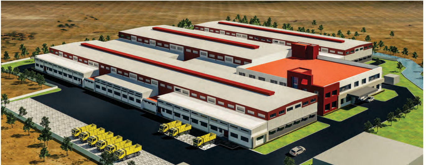
Autotex Plant II
